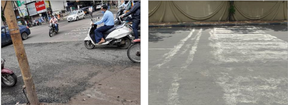
Figure 3: Bad or missing markings (left, 0 points), just OK markings (right, 1 point)
