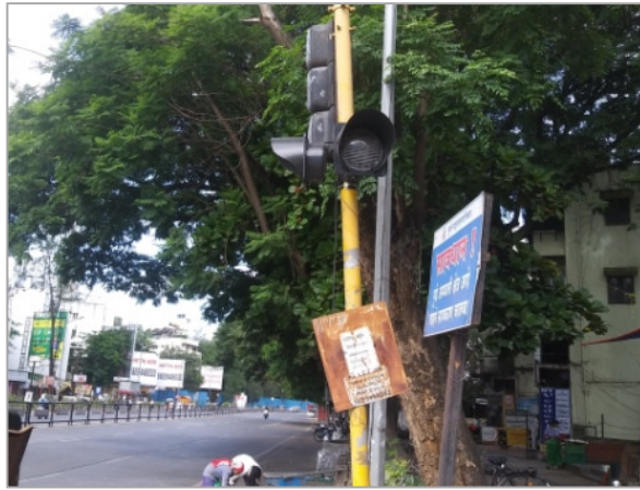
Figure 5: Non-functional pedestrian signal
